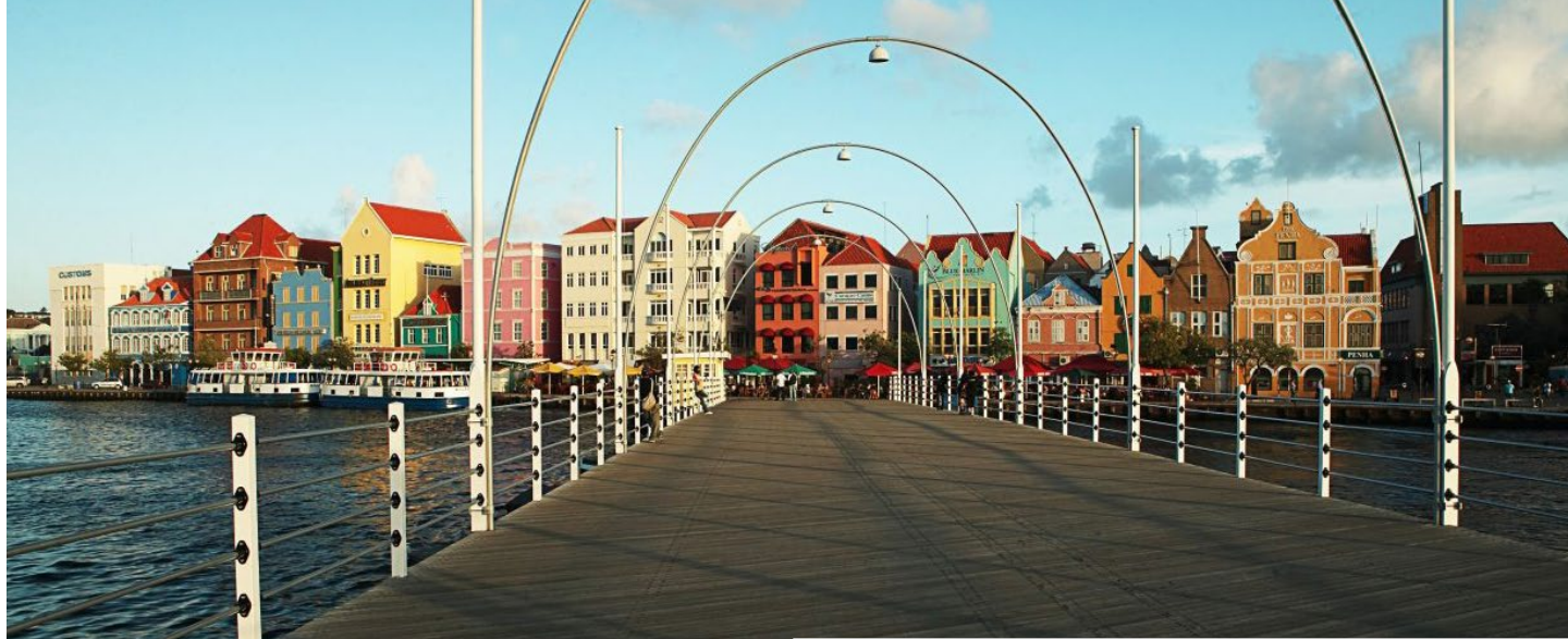
Queen Emma Swing Bridge in historic downtown Willemstad.
